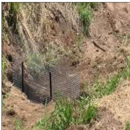
Left and Middle: Installation of DIY gabion, Right: Established gabion post weather event
